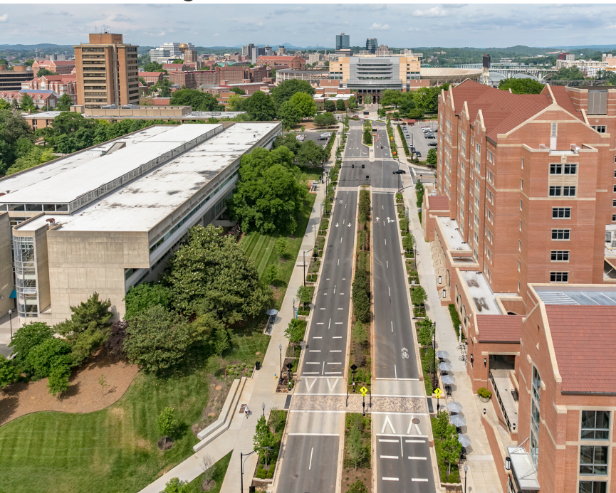
Bioswales lining Volunteer Boulevard
